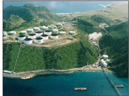
St. Eustatius Terminal – 13.0 mm bbls storage capacity
